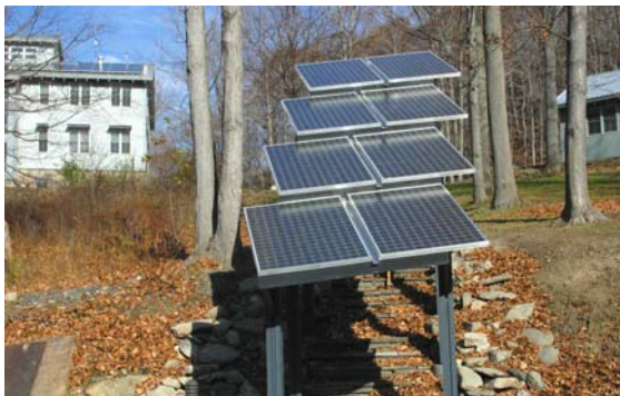
Solar panel roof over steps from parking lot.
